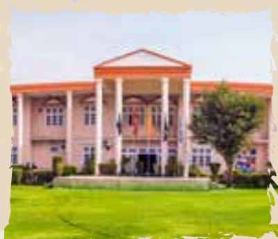
Frontier Campus Frontier Corps Building, Phase-6, Hayatabad, Peshawar Ph: (091) 5862977, 5861076
